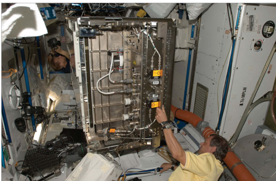
European Space Agency Astronaut Christer Fuglesang (left background) and NASA Astronaut Tim Kopra, both STS-128 mission specialists, install a Materials Science Research Rack-1 (MSRR-1) in the Destiny laboratory of the International Space Station.
